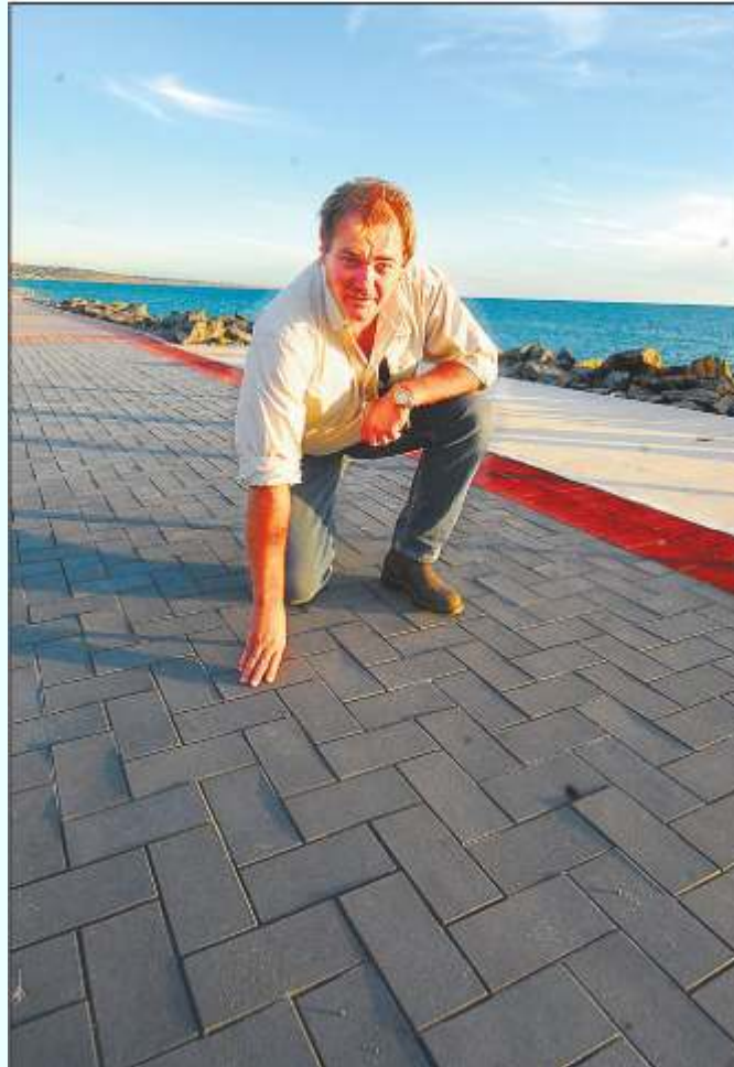
RECYCLED: Leon Immelman, from Enviropave Australia, with the pavers made from recycled car tyres. 103537
